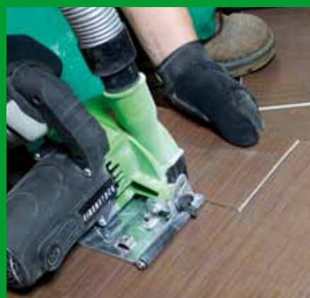
Cutting of tiles and cutouts in tiles
